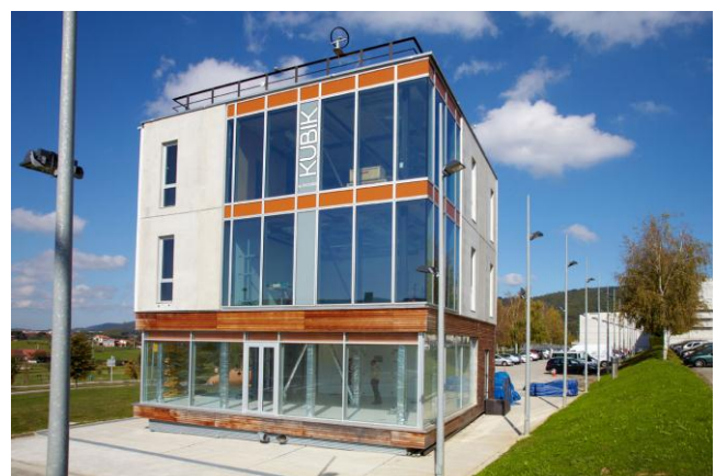
Figure 1. KUBIK building located in Zamudio, which has an advanced monitoring system; equipped with over 400 sensors that records conditions inside and outside the experimental facility.
